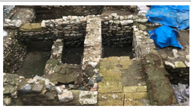
Figure 19. Algae formation on the horizontal surfaces of the walls.
