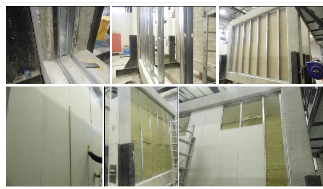
Figure 3. Gypsum Board Partition Wall Systems Manufactured at TSE.
