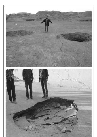
**Figure 8**. Ground voids and tension cracks formed after the collapse of a shallow qunat in Iran after the earthquake (Pellet et al., 2005).
