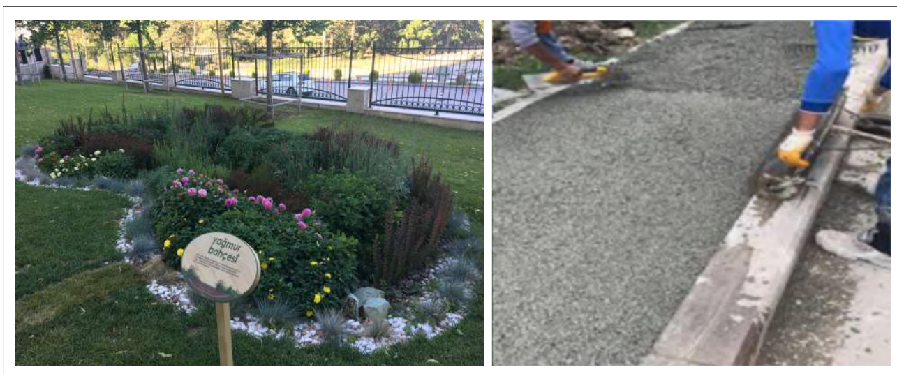
Figure 2. The implementation of permeable concrete and rain garden.
