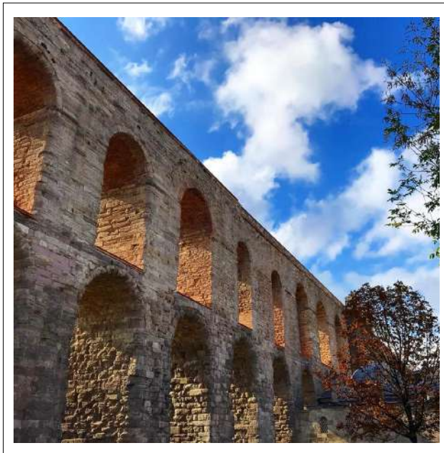
Figure 2. Bozdoğan (Valens) Aqueduct.
