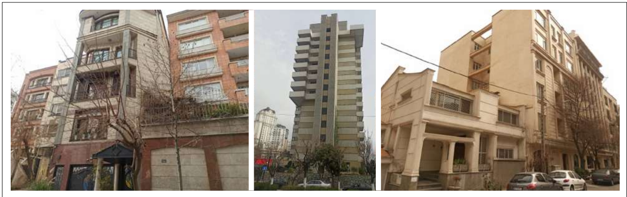
Figure 5. Facade/view, and city/ building interface of Tehran, Iran.
