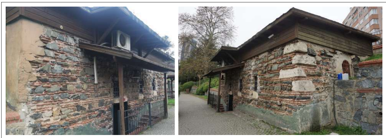
Figure 14. The existing structure of B4.
