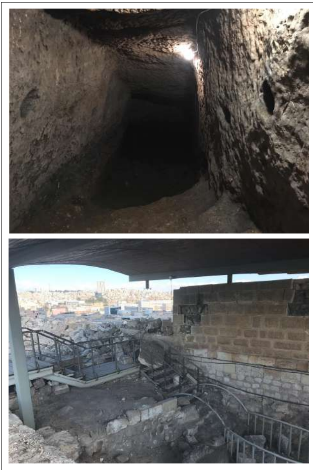
Figure 7. Gaziantep Castle tunnels lead to the bitter water-freshwater junction, and on the right, the view of the hill leading to the castle corridors after the earthquake (Umut Almaç 3 ).
