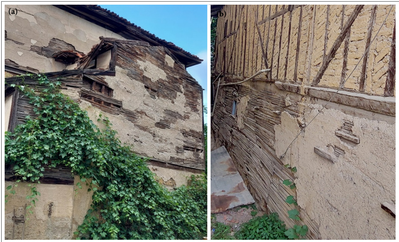
Figure 2. (a) Bağdadi system technique (Sinop) (b) Bağdadi and half-timbered system technique (Sinop).
