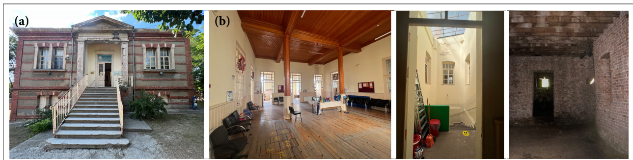
Figure 23. (a) Views from the east; (b) Timber structure of the Sofa , Additional staircase covered with skylight, wooden ceiling at basement floor.
