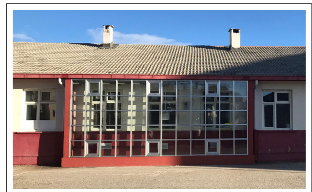
Figure 6. Applied second glass façade.
