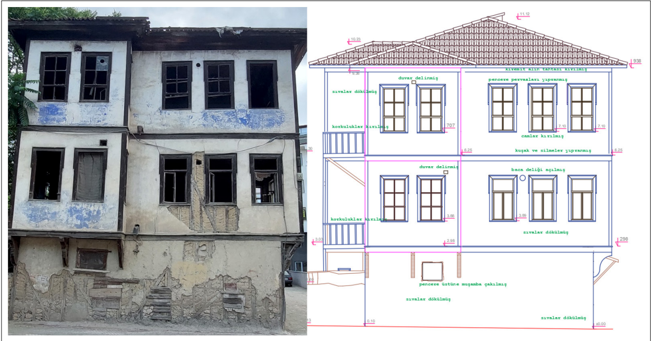
Figure 10. North facade of Mehmet Kaya House.
