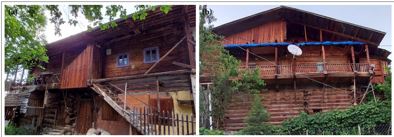
Figure 1. (a, b) Examples of timber structural systems created by sequential alignment of planks and logs Artvin/Türkiye.
