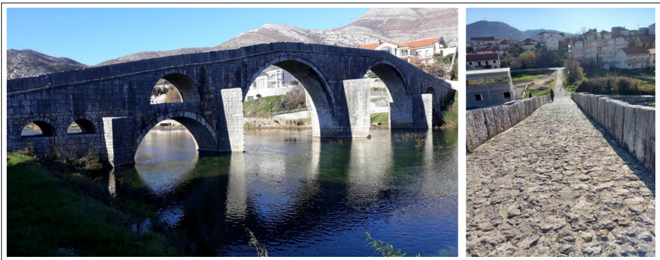
Figure 3. Arslanagić bridge in Trebinje after relocation, eastern upstream façade and paving (the photos were taken by the authors in 2022).
